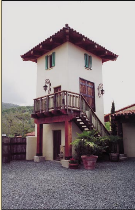
Biodynamic tower at the Ceàgo estate houses a cellar at the base to store biodynamic preparations and stirring tank in upper level to mix preparations and gravity feed the solutions to containers for spraying in the vineyard.
